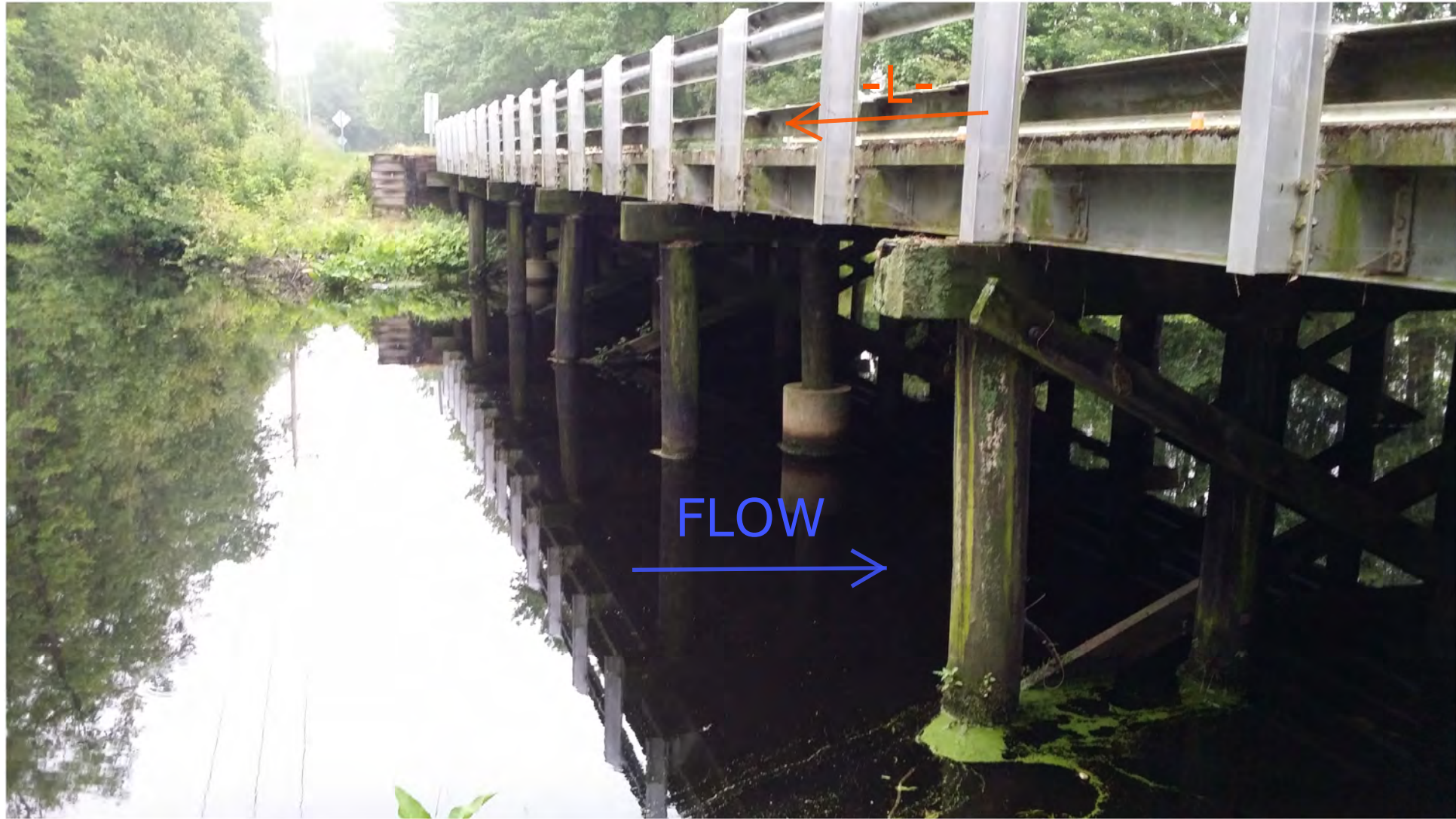
VIEW LOOKING EAST FROM END BENT 1
